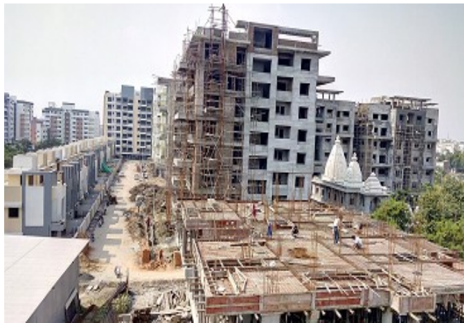
SFRC Internal Road for Housing Colony in Wathoda
