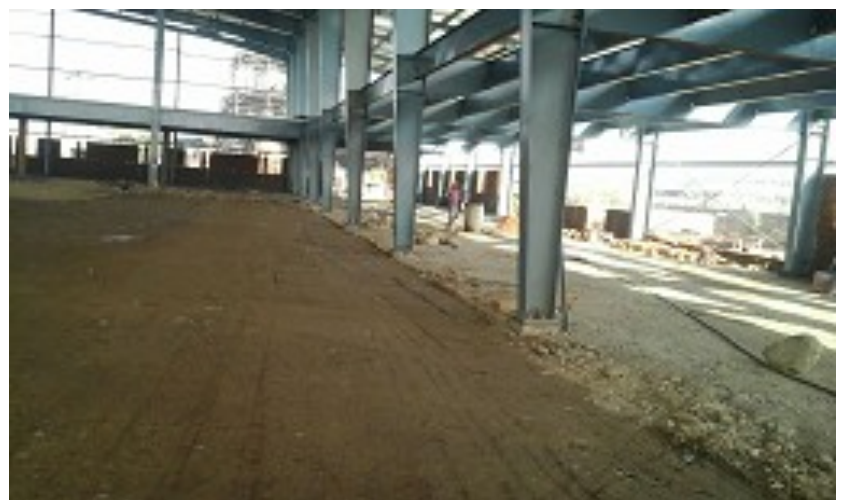
Casting of SFRC Flooring in Process (Right)
