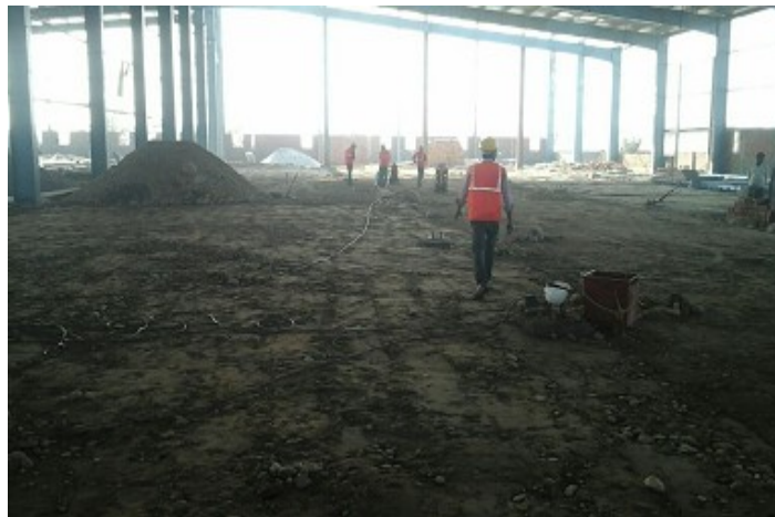
Ground Preparation for Warehouse Flooring (Above).
