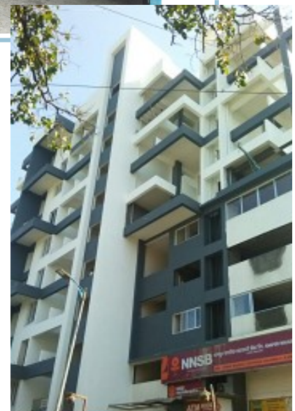
5,000 sq. ft. area has used Shaktiman Steel Fibres for Reinforcement (Above).
