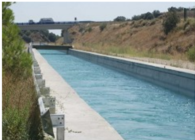
Lift Irrigation Canal (Right)
