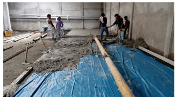
SHAKTIMAN® MSCF 50 was used with Tremix Technology
