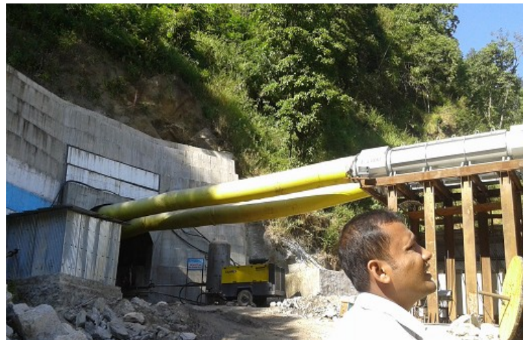
Entrance to the HEPP Tunnel (Right)
