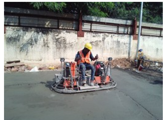
Finishing in progress at construction site
