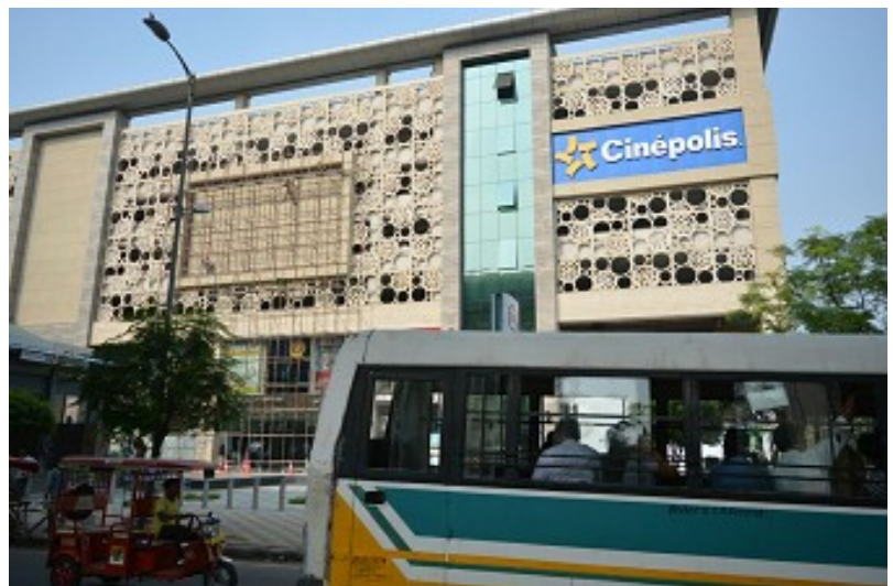
Rohini West Metro Station Parking Area (Right)
