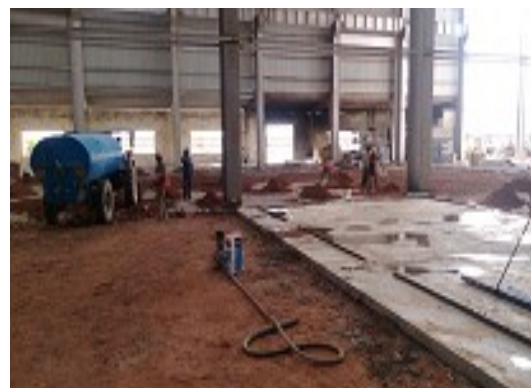
Casting in progress at construction site
